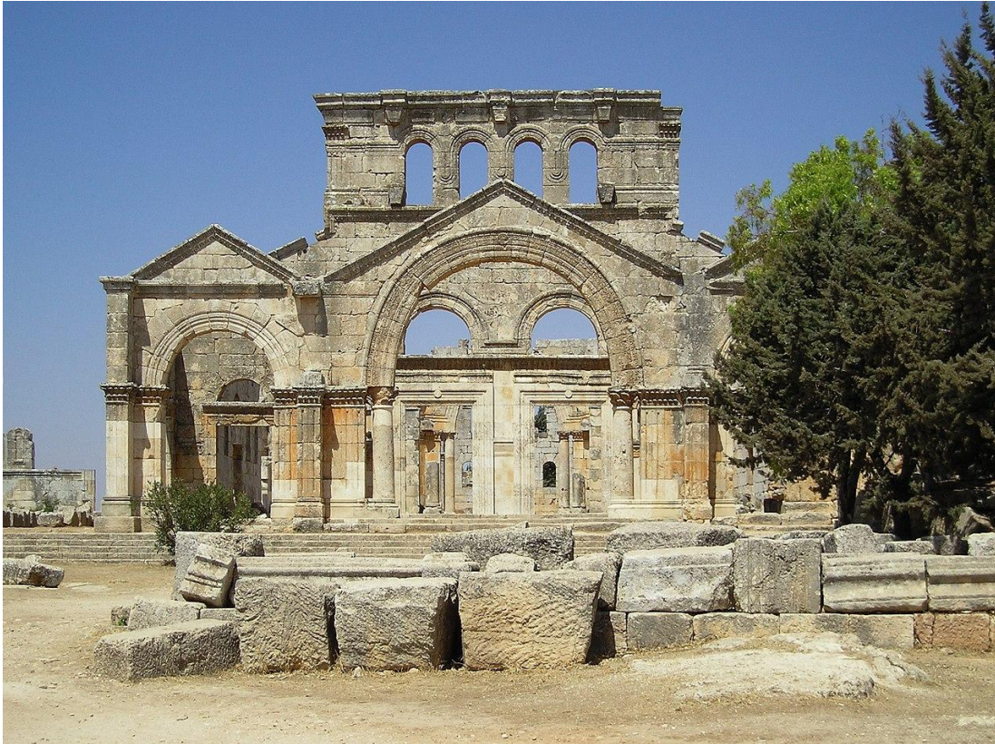
Figure 20: Main entrance (south basilica) of the Church of St. Simeon Stylites in Qal 'at Sim 'ān. The narthex had the form of an open porch with three connected portal houses. It is opened to the nave through four doors (in the background).
