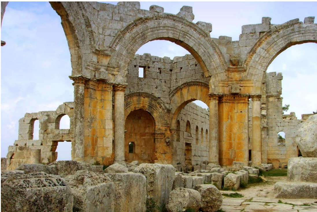
Figure 27: View from the central octagon of the Church of St. Simeon Stylites to one of the corner rooms containing an apsidiole. The corner rooms with apsidiole are equivalents of the squinches of other octagonal crossing towers.
