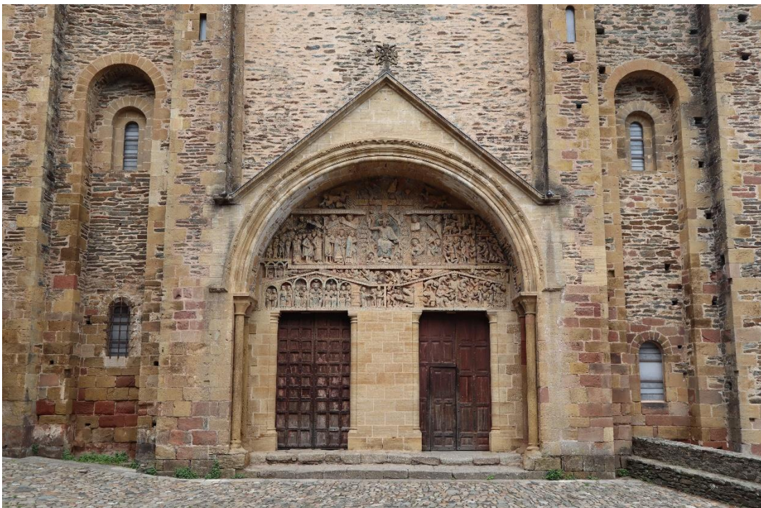
Figure 21: West portal of Sainte-Foy in Conques. The overall disposition with portal house, two widely separated entrance doors and blind portals to the left and to the right has no precedence in Romanesque architecture. It appears like a simplified version of the main entrance to the Church of St. Simeon Stylites in Qal 'at Sim 'ān.
