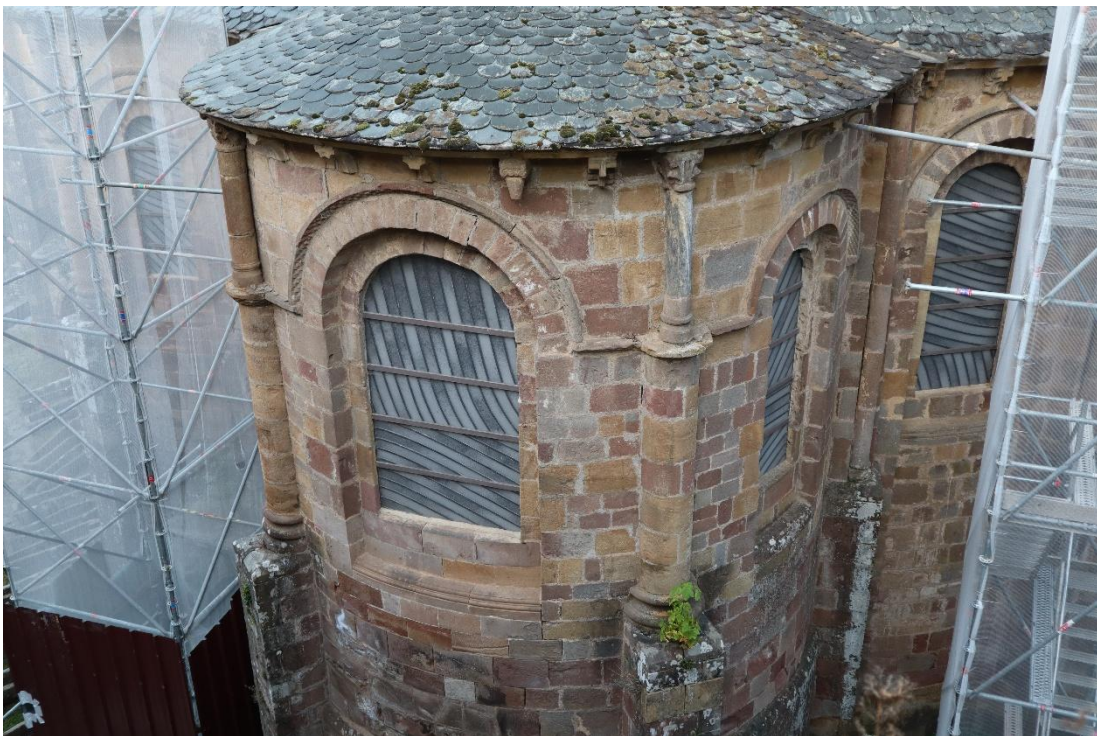
Figure 19: Radial chapel of Sainte-Foy in Conques looking like a height-compressed version of the central apse of the Church of St. Simeon Stylites. The size-reduced upper half-columns sit on the eyebrow shaped cornices of the windows rather than on a separate entablature above the windows.
