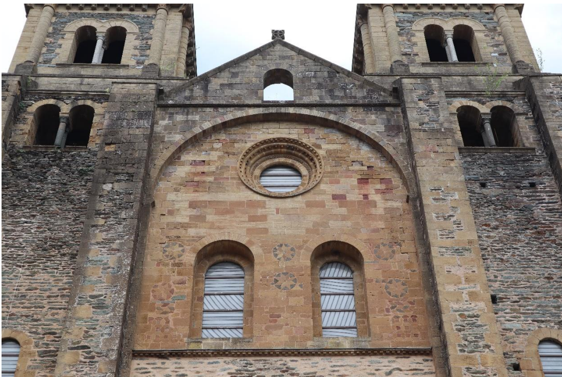
Figure 25: West façade of Sainte-Foy in Conques with its iconic framed grouped window. The transparent window at the top indicates that the steep gable has a purely decorative function. The roof of the nave has a significantly lower position than this gable. The two towers are fictitious reconstructions of the 19 th century.
