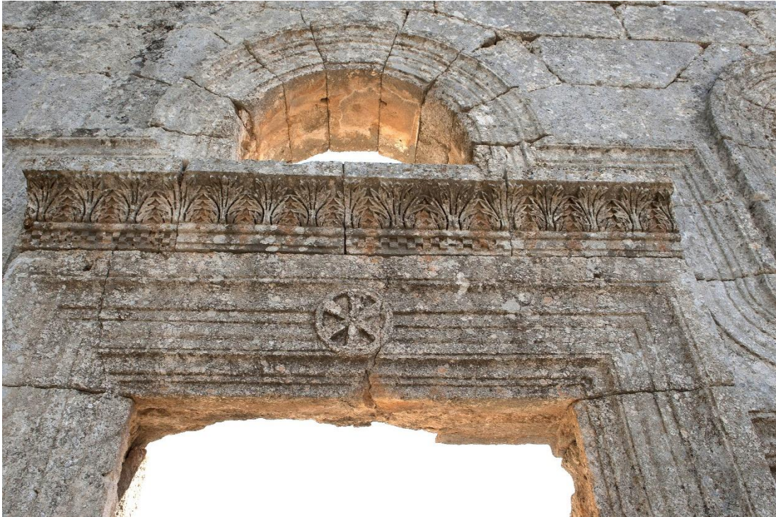
Figure 22: Portal of the north basilica of St. Simeon Stylites. The cornice above the door has double-row square billet moldings. The outer moldings of the cornice around the upper window have parallels with the portals of Conques.
