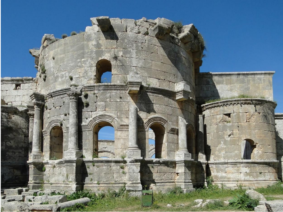
Figure 18: Central apse of the east basilica of the Church of St. Simeon Stylites in Qal 'at Sim 'ān. The apse had stacked columns on pedestals, separated by an entablature-like cornice. The windows have eyebrow shaped cornices.
