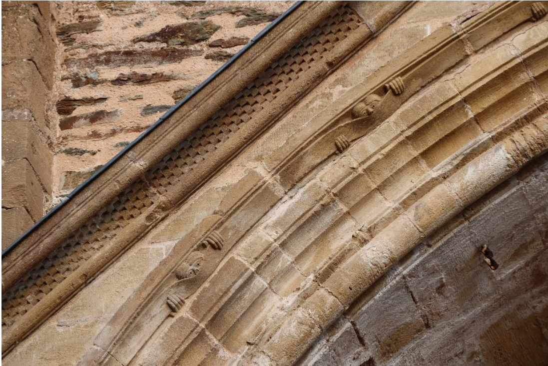
Figure 28: Archivolt of the west portal of Sainte-Foy in Conques. The moldings have significant structural similarity with corresponding moldings of the Church of St. Simeon Stylites. The reconstructed cornice of the portal house (upper left side) shows typical square billet moldings between two tori/rolls.
