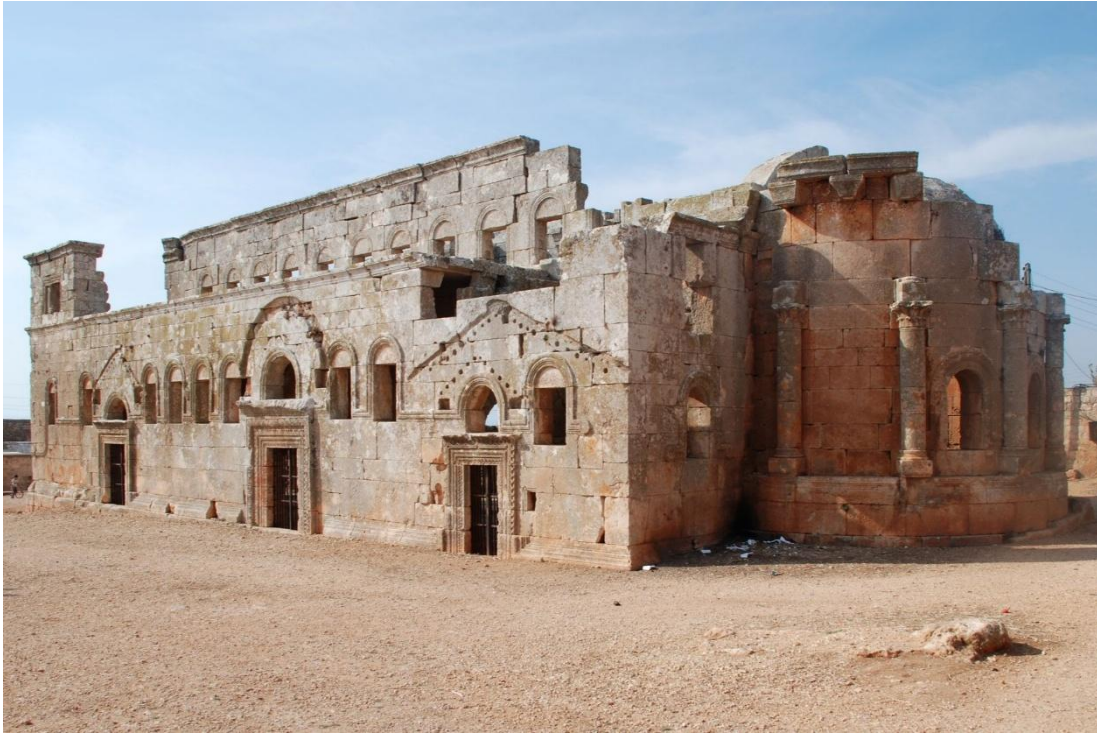
Figure 22: Basilica of Qalb Loze, dedicated to St. Simeon Stylites, which served as prototype for Qal ‘at Sim ‘ān. The apse (right) had stacked engaged columns. The cornices around the windows of the nave became characteristic features of the 6 th century architecture of North Syria.
