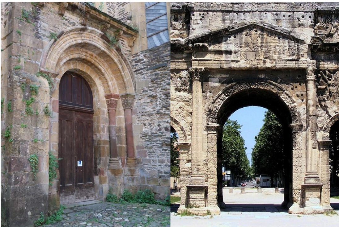
Figure 94: Portal of the northern transept of Sainte-Foy in Conques (left) and Roman triumphal arch in Orange (right). Most Roman triumphal arches do not feature the kind of pilasters under the archivolt that can be seen in Orange.
