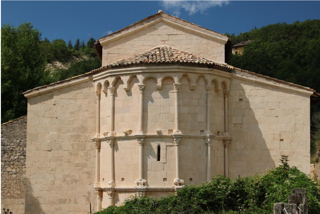
Figure 101: Apse of Santa Maria in Valle Porclaneta. The apse has stacked engaged columns and a roof cornice with a Lombard band, closely resembling the central apse of the east basilica of Qal 'at Sim 'ān.
