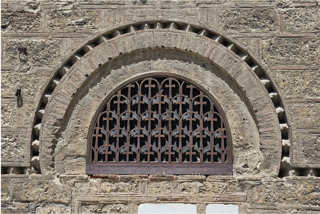
Figure 91: Lunette of the walled-up south portal of Panagia Kapnikarea in Athens. The cornice of the archivolt has the shape of a horseshoe arch, a typical element of the architecture of North Syria.
