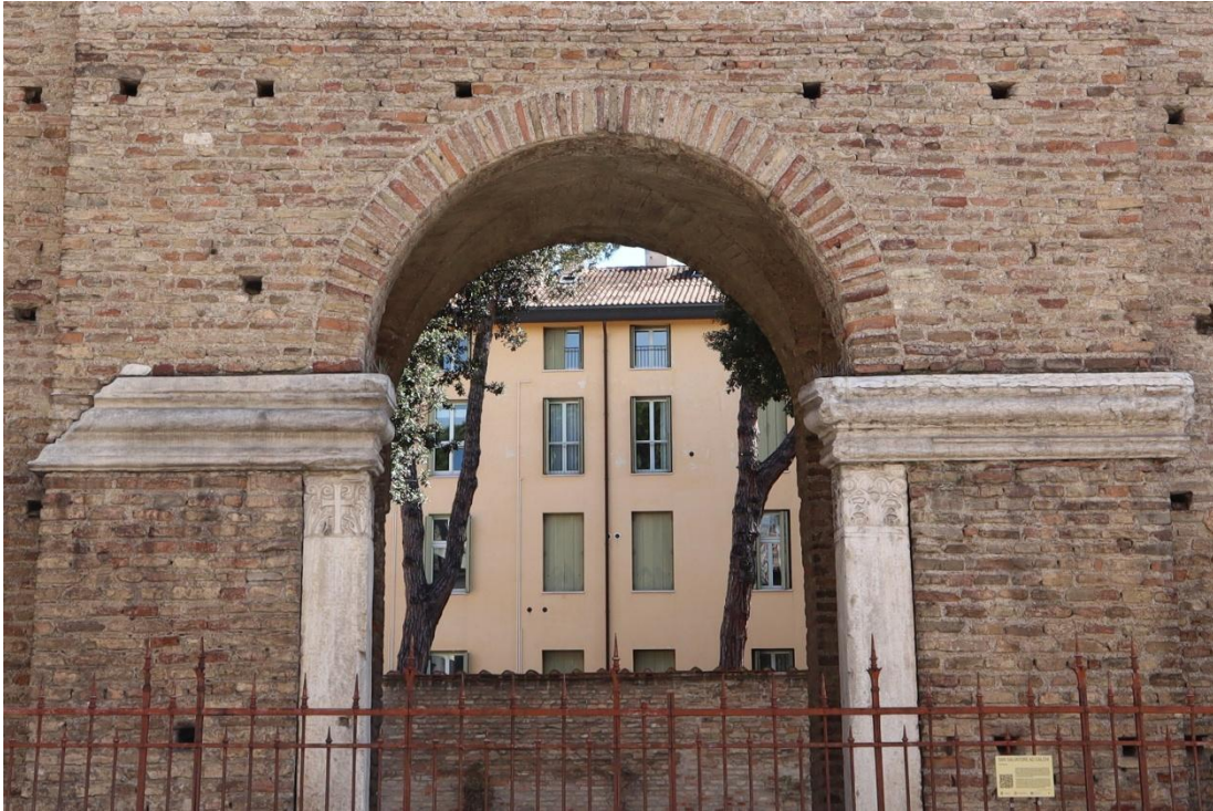
Figure 87: Palace Gate of the so-called Palace of Theoderic in Ravenna (6 th century). The horizontal cornices mimic a Syrian arch and are decorated with tori and scotiae. The Palace Gate itself followed the model of the Golden Gate of Diocletian's Palace in Split or the Chalke of the Great Palace in Constantinople (no longer extant).
