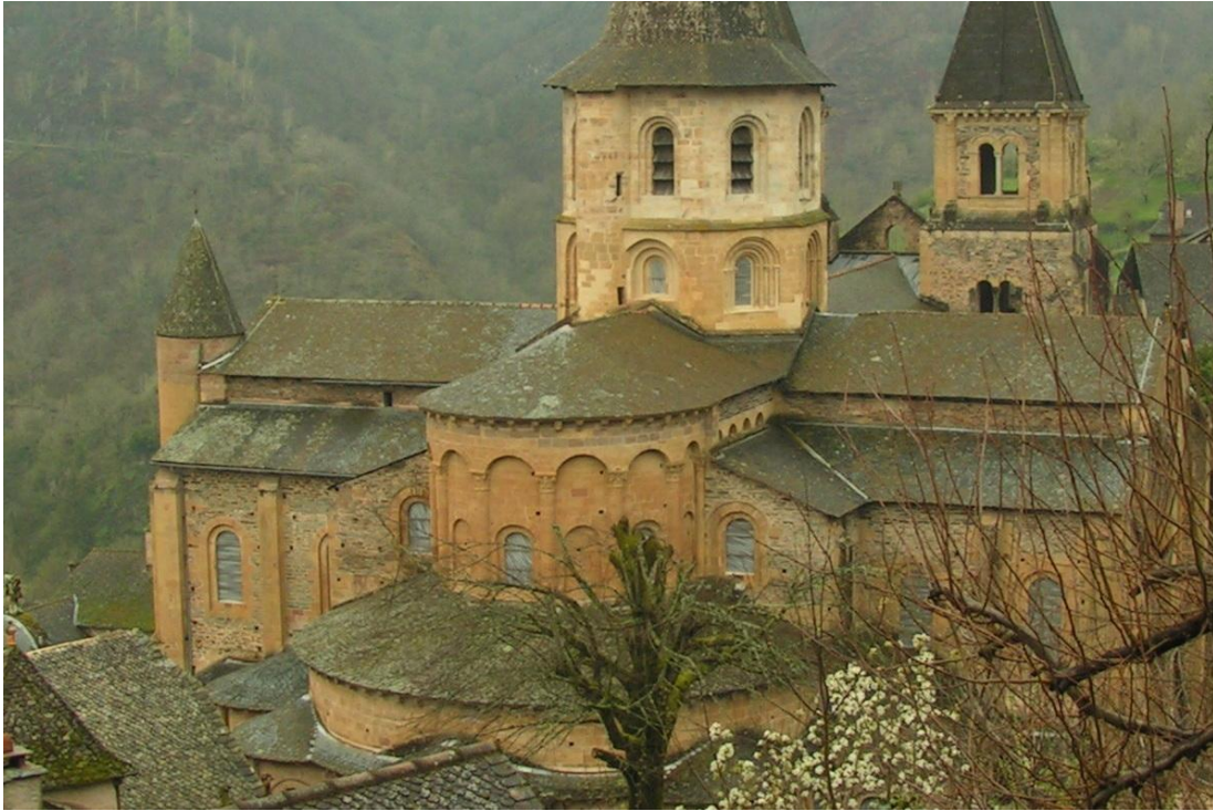
Figure 42: Chevet and crossing tower of Sainte-Foy in Conques. The apse has a large blind arcade. The masonry of the staircase tower attached to the crossing tower is not consistent with the lower story of the tower.
