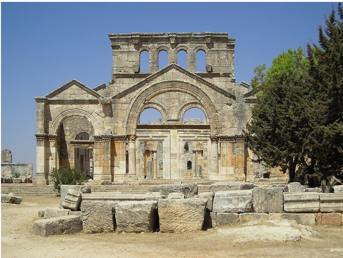
Figure 27: Main entrance (south basilica) of the Church of St. Simeon Stylites in Qal 'at Sim 'ān. The narthex had the form of an open porch with three connected portal houses. It is opened to the nave through four doors (in the background).
