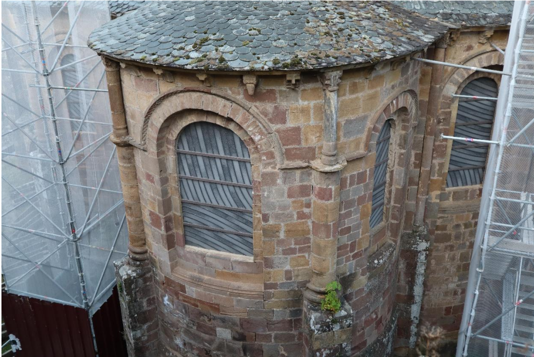
Figure 24: Radial chapel of Sainte-Foy in Conques, looking like a height-compressed version of the central apse of the Church of St. Simeon Stylites. The size-reduced upper half-columns sit on the eyebrow-shaped cornices of the windows rather than on a separate entablature above the windows.
