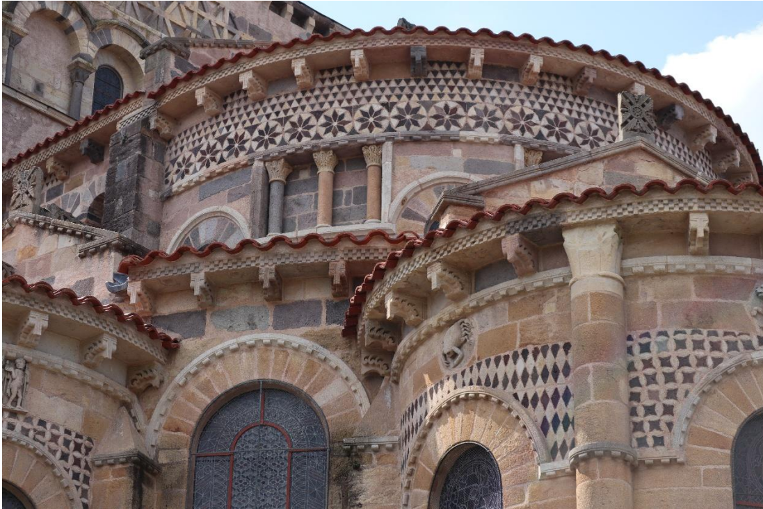
Figure 2: Chevet of Notre-Dame-du-Port in Clermont-Ferrand with typical decorative elements of the Romanesque architecture of the Loire, Burgundy, and Auvergne. These include square billet moldings and shaving consoles at the roof cornices as well as single-row round billet moldings at the eyebrow-shaped cornices around the windows. The black inlay patterns are a typical feature of Auvergne.
