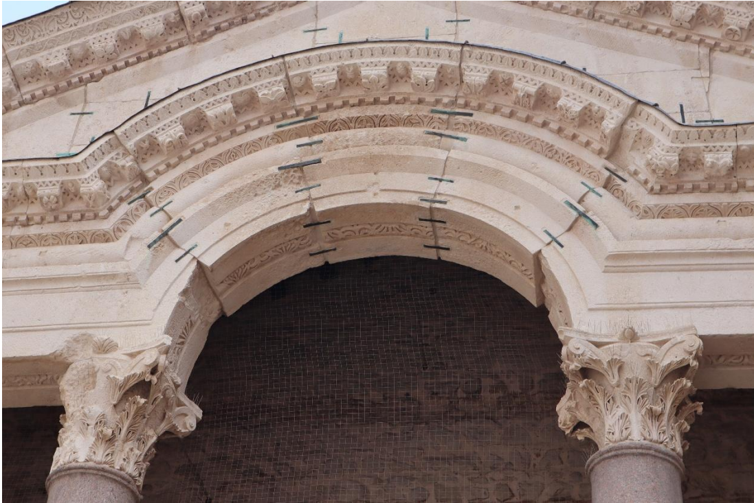
Figure 85: Syrian arch of the Peristyle of Diocletian's Palace in Split. The upper fascia of the archivolt is replaced by an Egyptian torus (here, more precisely: ovolo) and cavetto molding, following the 3 rd century architecture of Syria. The frieze consists mostly of dentils.
