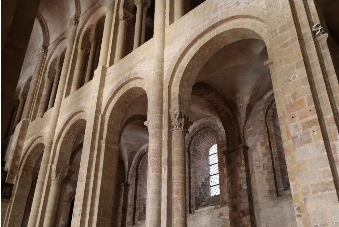
Figure 12: Northern arcade of the nave of Sainte-Foy in Conques. The image shows the four western bays of the nave, not including the fifth bay next to the crossing. The alternating supports at arcade level correspond to a pseudo-sequence of pier – column – pier – column – pier. At gallery level, the alternation has been suspended in favor of consistent half columns supporting the transverse arches of the vaulting.
