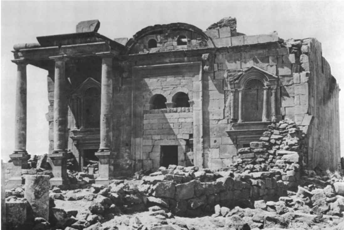
Figure 81: Roman temple of Mismiyeh (now destroyed) with an Egyptian torus frame around the central window and portal. The aedicula (right) is crowned by a Syrian arch with a torus between two cavetto moldings.
