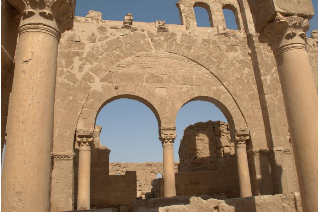
Figure 46: Mullioned portal with unusual outer engaged columns, inserted in the wide arcade of the Basilica A in Resafa.
