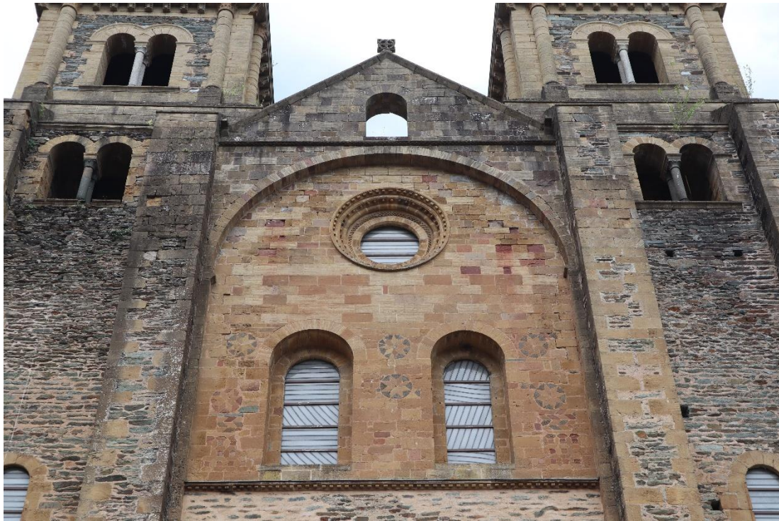
Figure 40: West façade of Sainte-Foy in Conques with its iconic framed group of windows. The transparent window at the top indicates that the steep gable has a purely decorative function. The roof of the nave has a significantly lower position than indicated by this gable. The two towers are fictitious reconstructions from the 19 th century.
