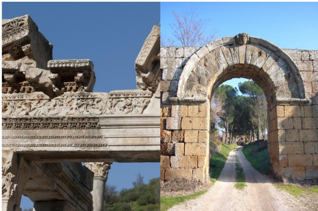
Figure 74: Entablature of the so-called Temple of Hadrian in Ephesus (left) and a city gate of Falerii Novi (right) exemplifying typical decoration elements of Graeco-Roman temples and of Roman Republican portals. The modern reconstruction of the right part of the entablature of Ephesus (left) clarifies its underlying geometrical structure.
