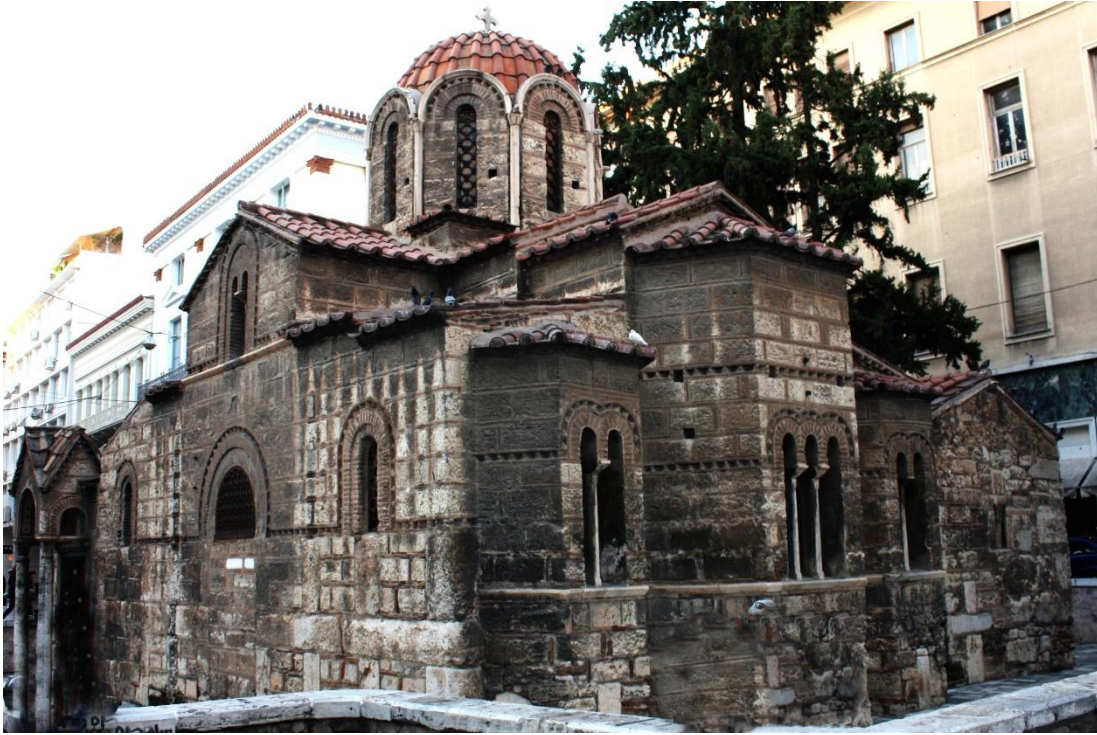
Figure 89: South façade and chevet of Panagia Kapnikarea in Athens. The eyebrow-shaped cornices of the windows of the apses and the fully framing cornices of the windows of the south façade replicate the equivalent cornices of the Church of St. Simeon Stylites in Qal 'at Sim 'ān and of other North Syrian churches, such as Qalb Loze.
