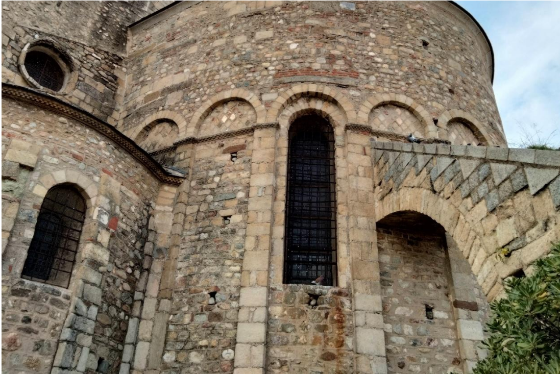
Figure 99: Apse of the cathedral of Elne from the middle of the 11 th century. The buttress on the right side is a later addition. According to a historic source, the apse was built after the model of the Anastasis in Jerusalem.
