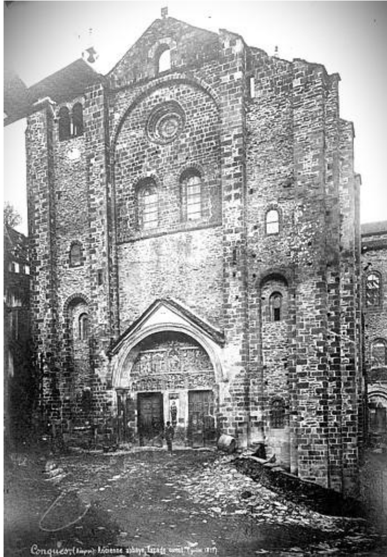
Figure 56: West façade of Sainte-Foy in Conques in its condition before the restoration of 1877. Today's massive double towers do not yet exist. The northwestern corner has a turret that hardly breaks through the silhouette of the gable. It has been speculated that a second turret may have existed at the southwestern corner but may have been destroyed in 1586, during the Wars of Religion. However, there is no proof for the former existence of a second turret. Like today, the gable has a decorative function and does not support the roof.
