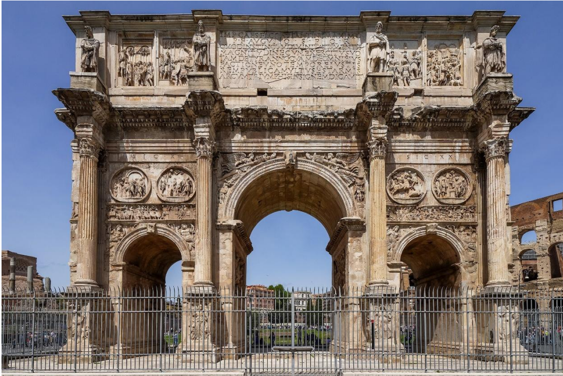
Figure 93: Arch of Constantine (315) in Rome. The archivolts of the three portals have cavetto cornices and three fasciae with astragals, following the traditional Graeco-Roman model. The archivolts are not supported by columns or pilasters.
