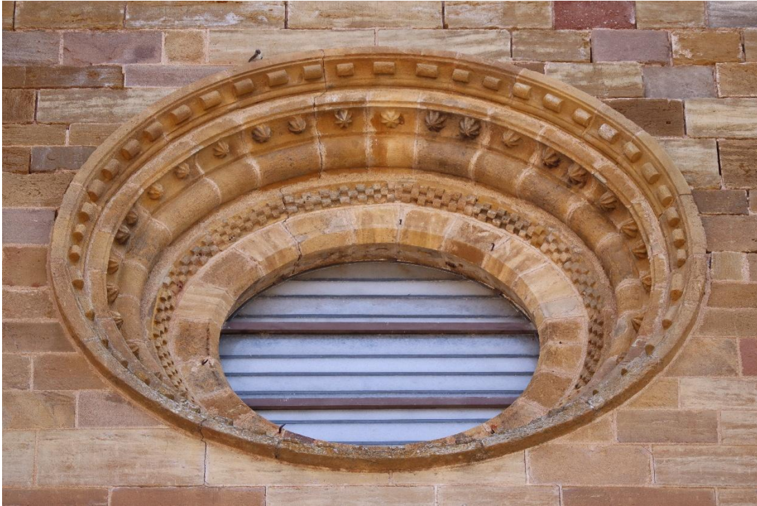
Figure 38: Modern reconstruction of the large oculus of the west façade of Sainte-Foy in Conques.
