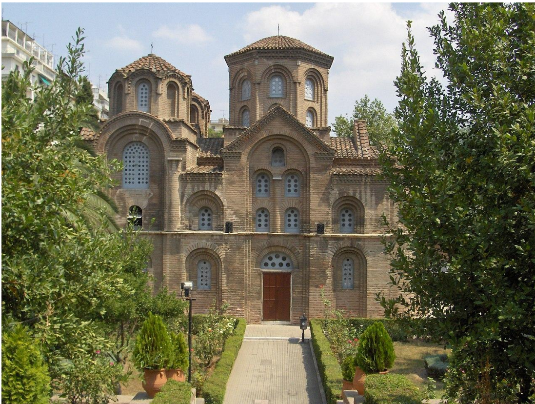
Figure 51: South façade of Panagia Chalkeon in Thessaloniki. The stepped frames around the windows are characteristic innovative features. The frame around the five windows of the transept has high similarity to the framed group of windows of the west façade of Conques. The decorative gable of the transept was unusual in Byzantine architecture.
