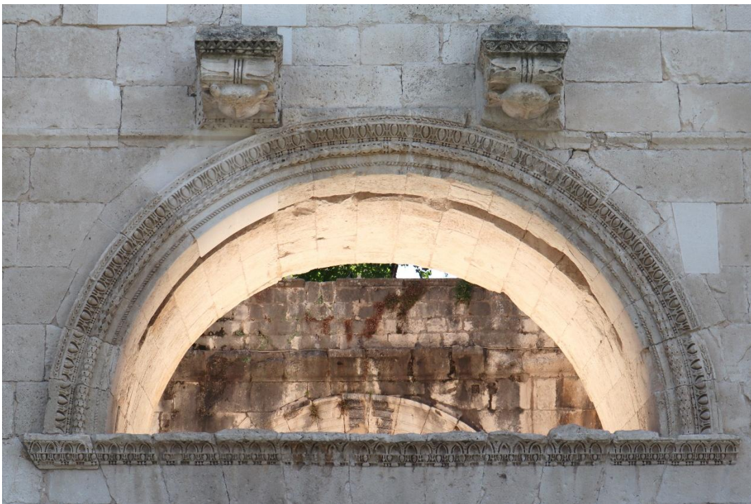
Figure 86: Archivolt of a lunette at the Golden Gate of Diocletian's Palace in Split. The archivolt follows the example of Hauran with a decorated cavetto cornice, a decorated torus, and two fasciae with an astragal. The general structural is similar to the architrave of the Peristyle of Split and the archivolt of Kfar Bar'am.
