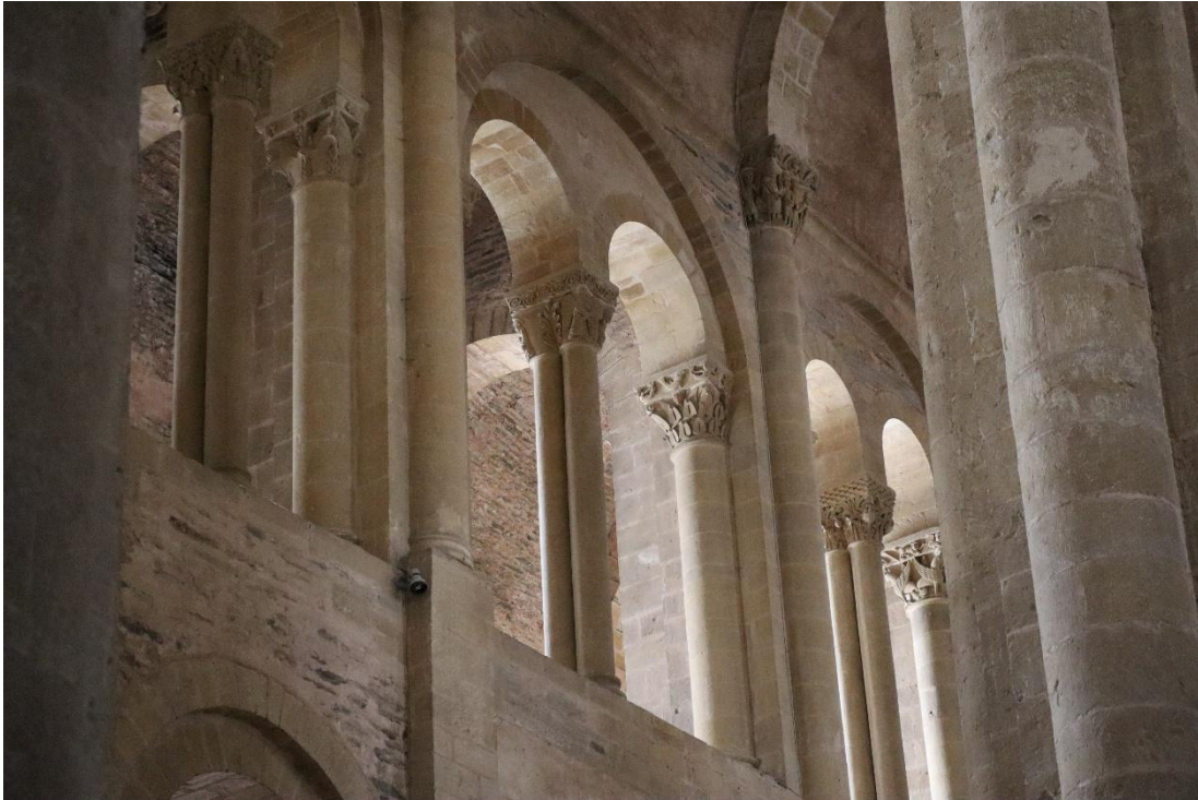
Figure 44: Southern gallery of the nave of Sainte-Foy in Conques. The mullioned windows have coupled columns at the center and additional outer half columns. The outer half columns are a frequent feature of French Romanesque architecture. They have no earlier correspondence in Roman architecture.
