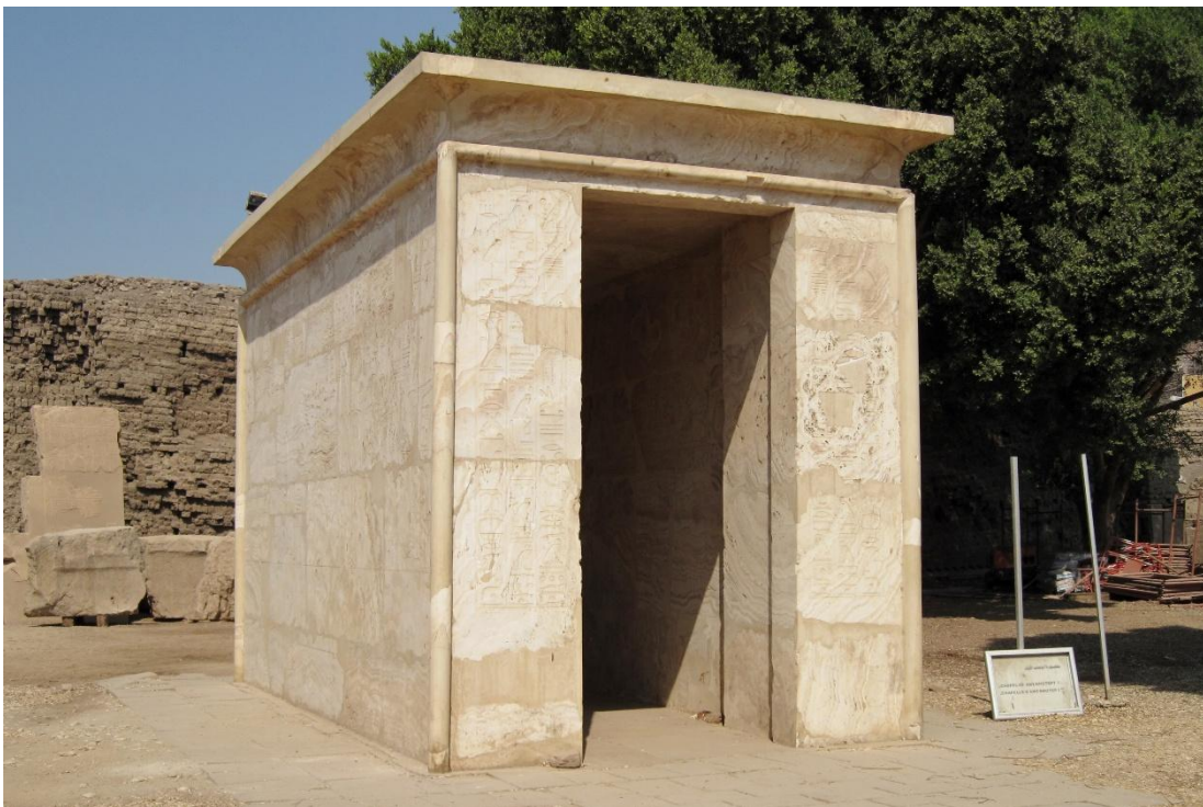
Figure 76: Alabaster chapel in Karnak with the typical ornamental elements of traditional Egyptian temples: cavetto cornice and tori (more precisely: rolls), the latter emphasizing the edges of the building.
