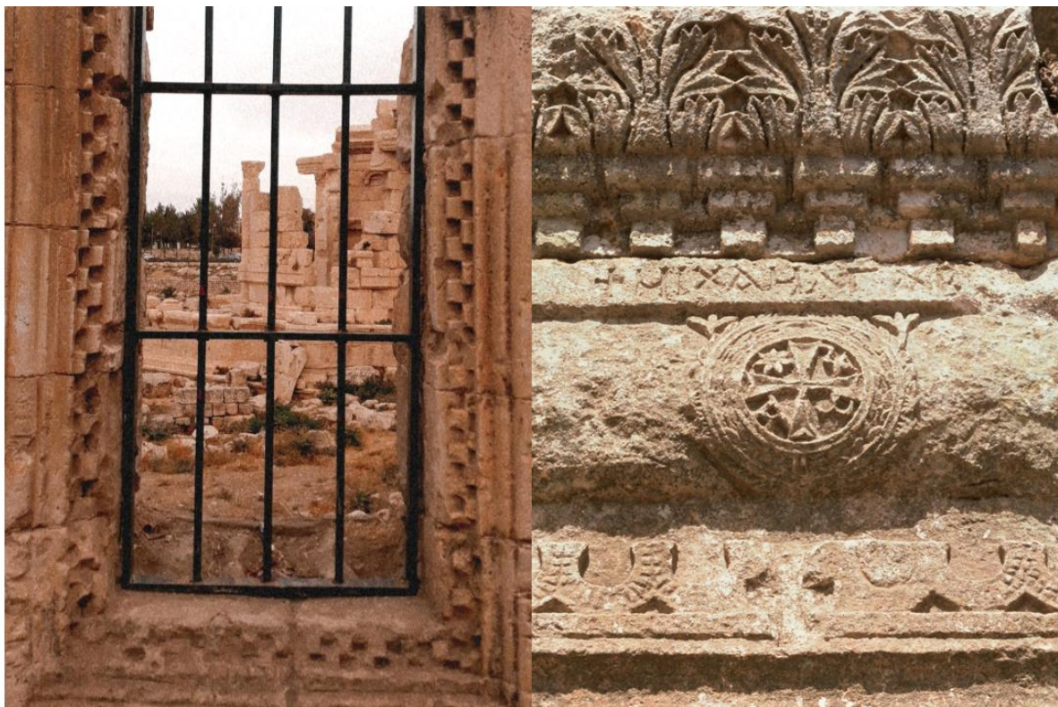
Figure 33: Multi-row dentils at a ruined window next to the so-called Temple of Venus in Baalbek (left) and at the central portal of the south façade of Qalb Loze (right).
