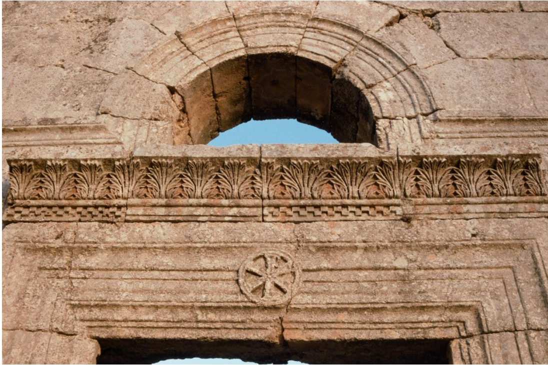
Figure 32: Portal of the north basilica of St. Simeon Stylites. The cornice above the lintel has double-row dentils.
