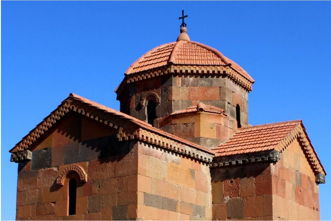
Figure 34: Partially reconstructed roof cornices with double-row dentils of the church of S. Astvatsatsin, next to the cathedral of Talin in Armenia. The window on the left is framed by an eyebrow-shaped cornice.
