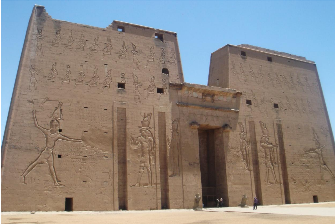
Figure 75: Pylon of the Ptolemaic Temple of Edfu. The central portal has a cavetto cornice. The edges of the pylon are decorated with tori. In Ptolemaic times, cavetto cornices and tori also were used at architraves of colonnades.
