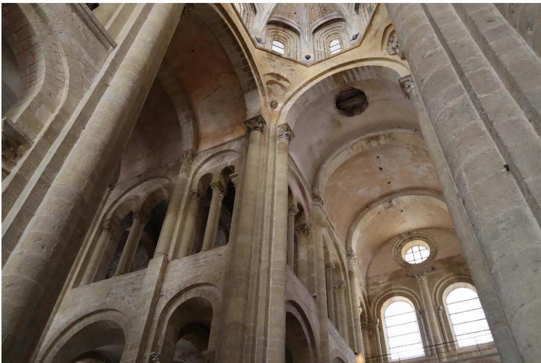
Figure 13: Galleries of the nave (left) and the northern transept (right) of Sainte-Foy in Conques. The first narrow bay of the nave has a parallel in St. John of Ephesus. Like in Ephesus, the sequence of alternating supports starts with its first pier only after the compound pier of the crossing, as is visible from the pilaster strip at arcade level. This disposition may have mimicked the massive quadrupedal piers of the crossing of Ephesus.
