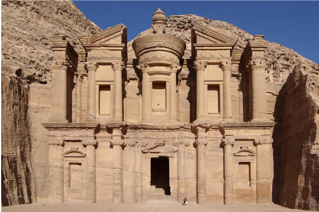
Figure 77: Tomb Ed-Deir in Petra as an example of Ptolemaic architecture with broken pediment, broken and curved entablatures, and aediculae in the façade. The cornices of its precursor Al-Kazneh already show first convex moldings.
