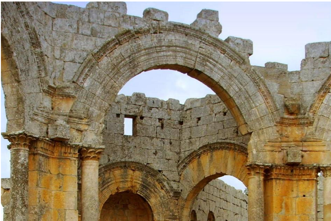
Figure 31: View from the central octagon of the Church of St. Simeon Stylites to one of the corner chapels with an apsidiole. The corner chapels with apsidiole are equivalents of the squinches of other octagonal crossing towers.
