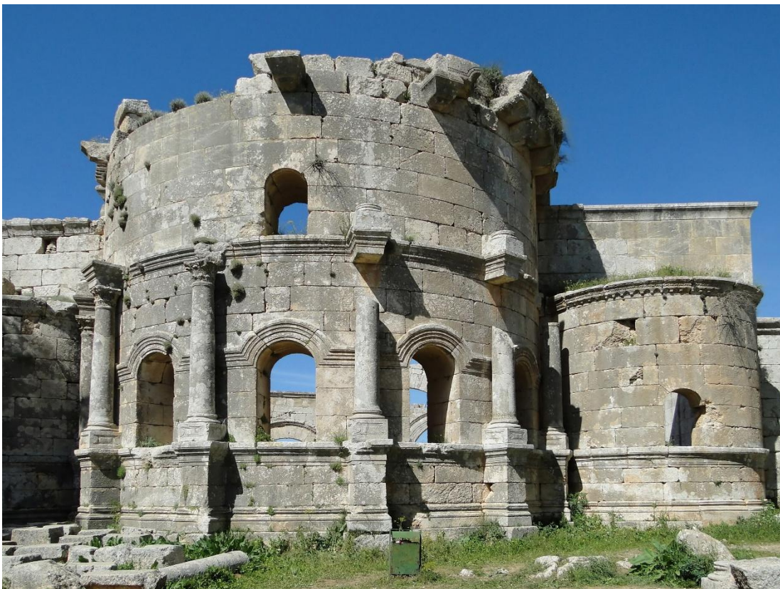
Figure 25: Central apse of the east basilica of the Church of St. Simeon Stylites in Qal 'at Sim 'ān. The apse had stacked columns on pedestals, separated by an entablature-like cornice. The windows have eyebrow-shaped cornices.
