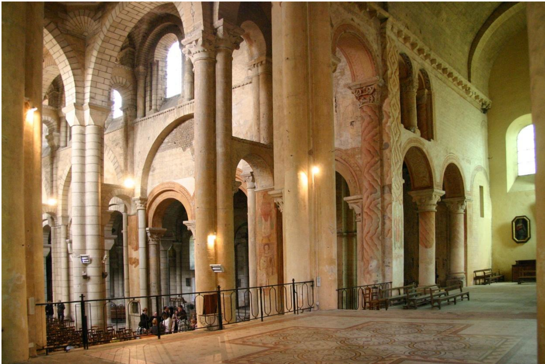
Figure 15: First bay of the nave and northern transept of Saint-Hilaire-le-Grand in Poitiers in its current condition. The domes of the nave, of which only one squinch is visible (upper left corner), are reconstructions of the 19 th century.
