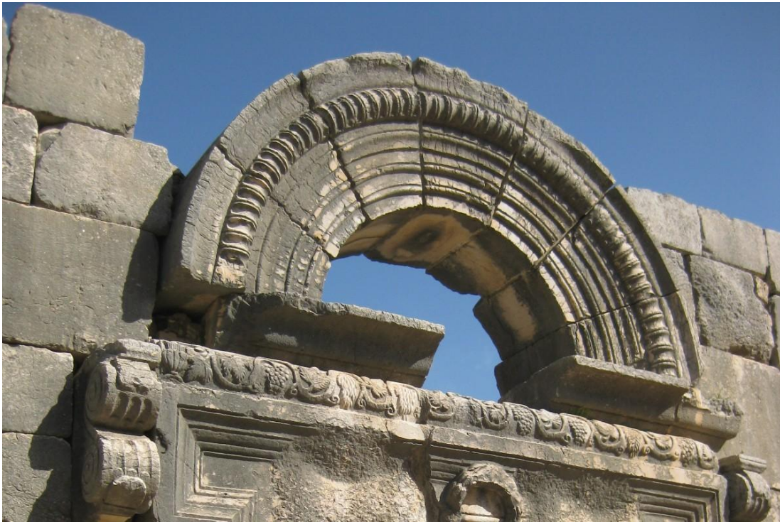
Figure 82: Portal of the synagogue Kfar Bar'am. This prototypical archivolt is a fusion of elements of Roman Republican (cavetto cornice), Egyptian (torus, fillet, and cavetto molding), and Greek (three fasciae with astragals) architecture.
