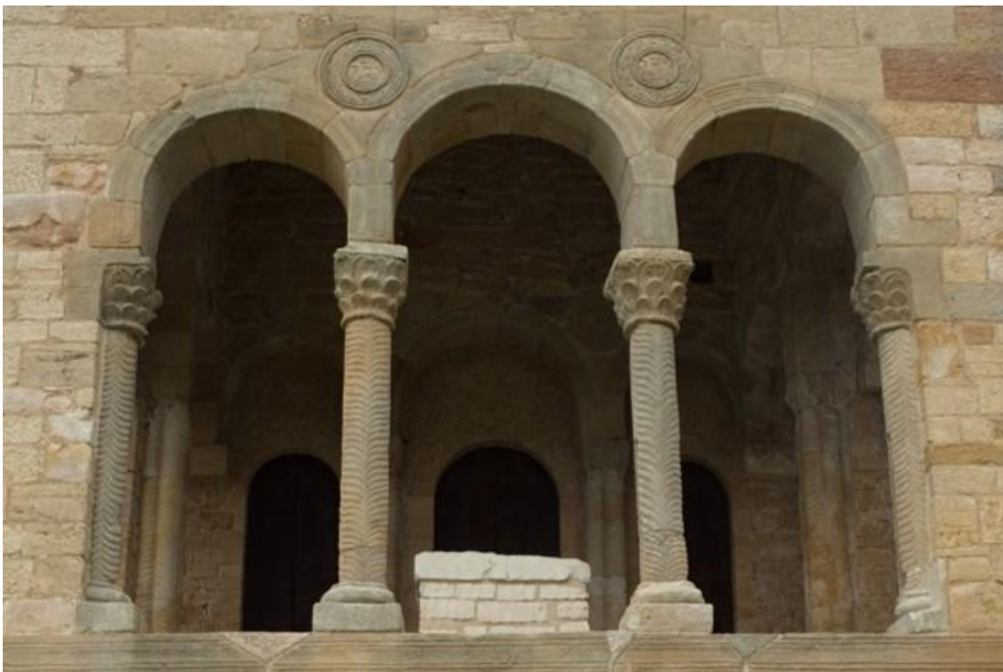
Figure 47: Mullioned window of the east façade of Santa María del Naranco near Oviedo. The window has unusual outer engaged half columns. The overstretched arches point towards Byzantine origins.
