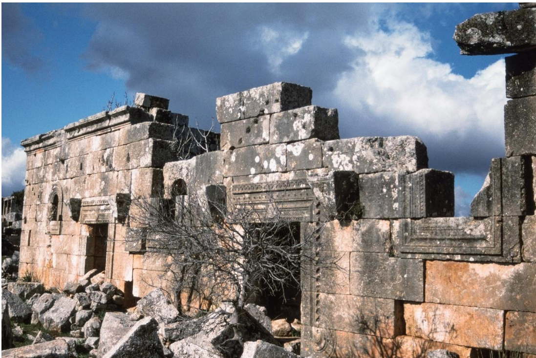
Figure 39: Ruins of the East Church of Qal 'at Kalota near Qal 'at Sim 'ān. The arched windows (left and right) were entirely framed by convex and concave moldings, deviating from common practices in North Syria.
