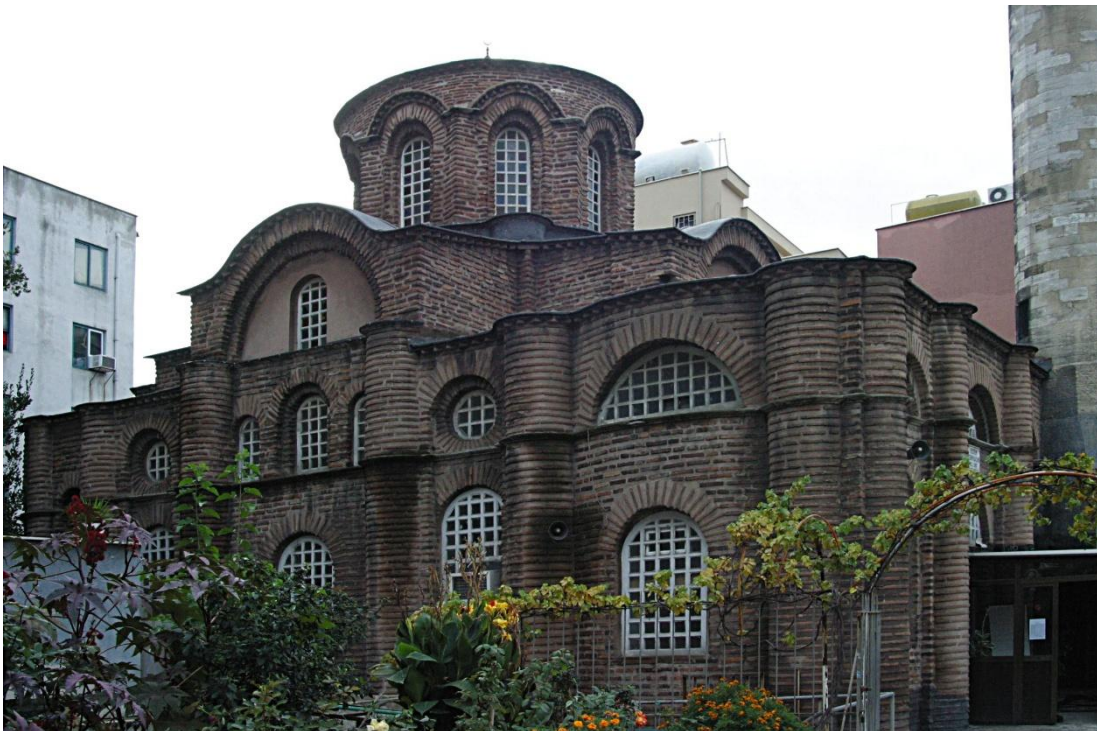
Figure 53: Myrelaion in Constantinople, one of the first cross-in-square churches incl. a single-story crossing tower.
