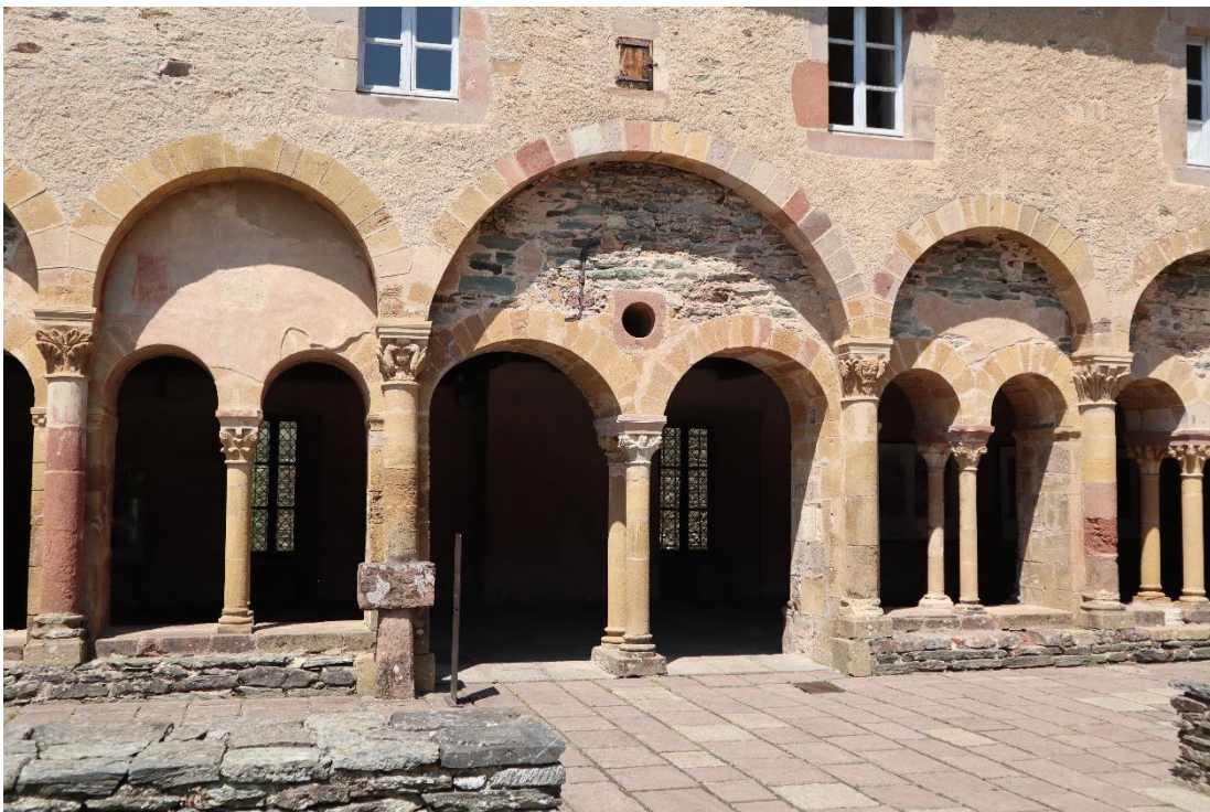
Figure 49: Portal and windows of the cloister of Sainte-Foy in Conques. The mullioned portal and windows have coupled columns. The mullioned portal has an oculus in the spandrel of its arches. The arcades of Hagia Sophia in Constantinople feature black circular inlays at the same low position. Such a low position is unique in Romanesque architecture.
