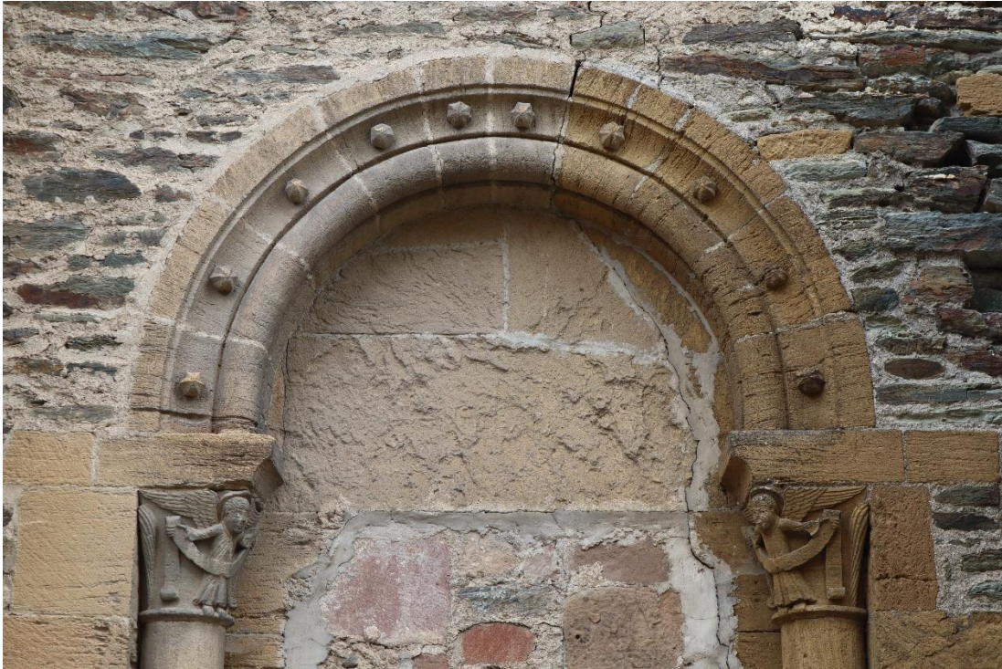
Figure 36: Walled-up south portal of Sainte-Foy in Conques. The structure of the archivolt is simplified compared to the other portals of Conques. Instead, the scotia of the archivolt is filled with ball-shaped stars.
