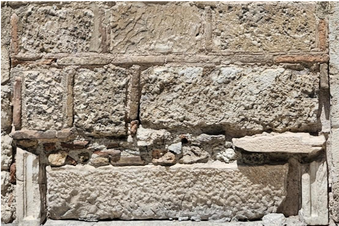
Figure 92: Relics (below left and right) of the jamb of the south portal of Panagia Kapnikarea in Athens, now walled up. The original jamb included tori at the edges and associated scotiae. This and other jambs of Athens are much closer to the decorative style of Syria than comparable 6 th century jambs of Constantinople or Ravenna.
