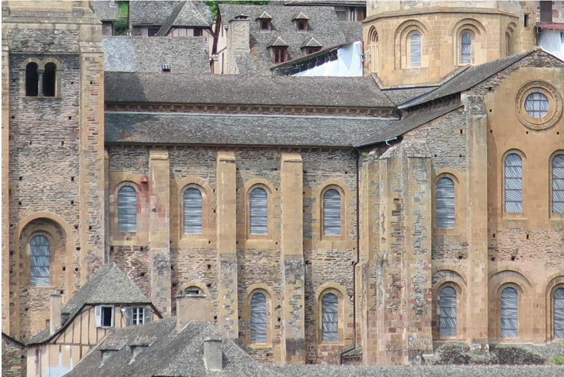
Figure 50: South façade of Sainte-Foy in Conques. The many stepped frames around the windows are clearly visible.
