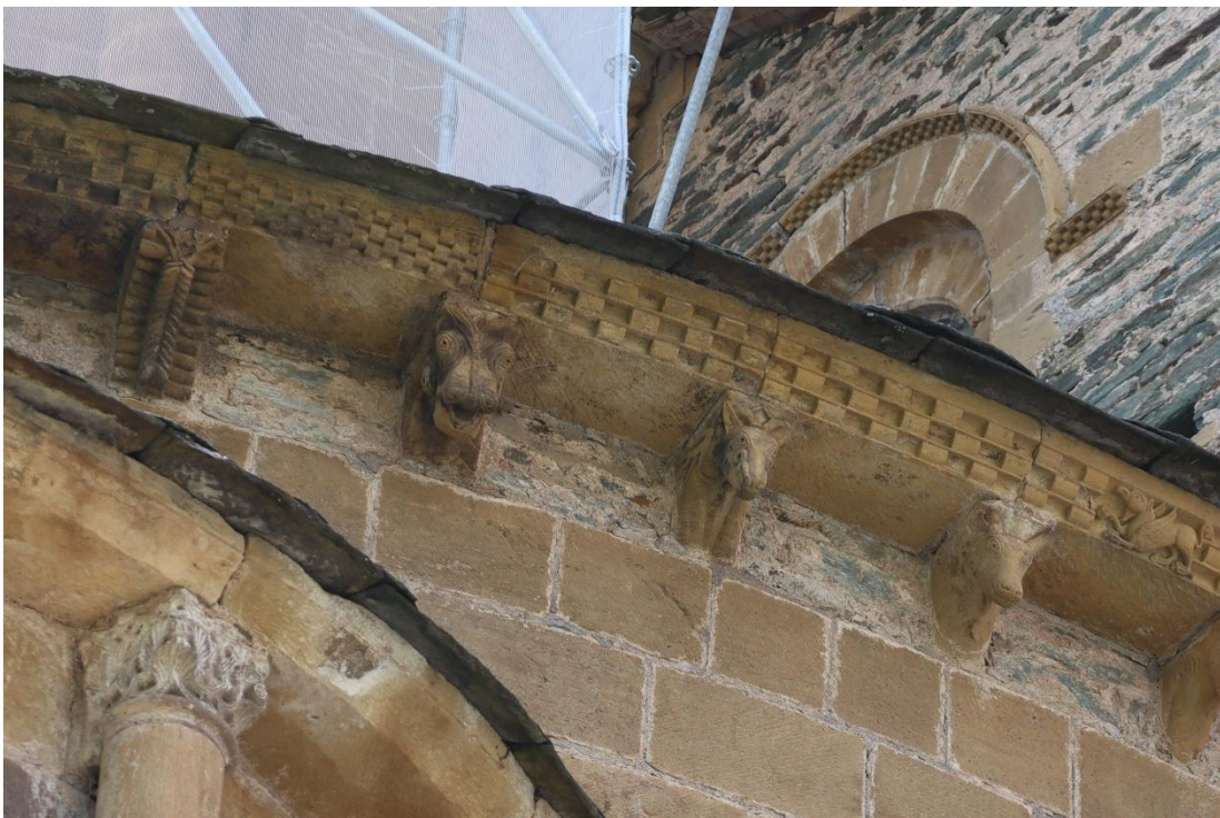
Figure 3: Cornices of the ambulatory and of a radial chapel of Sainte-Foy in Conques. The cornice of the ambulatory is decorated with the characteristic multi-row round billet moldings of Conques with separating lines between the rows of billets. The round billet moldings of the transept window above do no longer have these separating lines. Most of the consoles of the ambulatory have animal masks. The earlier shaving type can be seen on the left.
