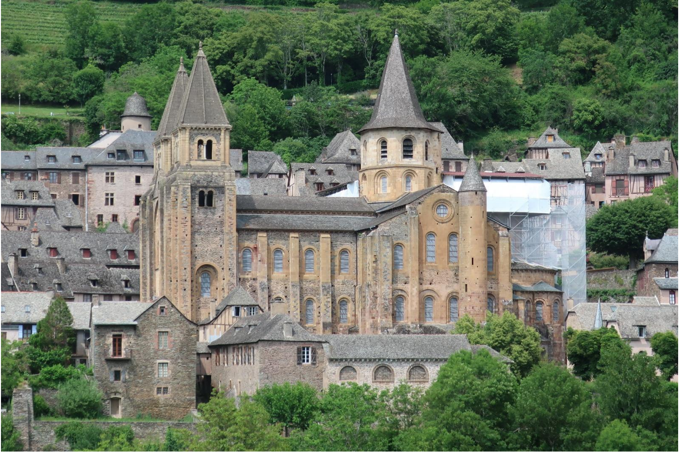
Figure 1: South façade of the abbey church of Sainte-Foy in Conques. The prominent west towers are fictitious reconstructions of the 19 th century. The second story of the crossing tower was added in the 15 th century. The apse with its blind arcade is hidden by the scaffolding.
