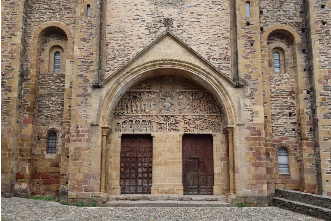
Figure 26: West portal of Sainte-Foy in Conques. The overall disposition with portal house, two widely separated entrance doors and blind portals to the left and to the right has no precedence in Romanesque architecture. It can be read as a simplified version of the main entrance to the Church of St. Simeon Stylites in Qal 'at Sim 'ān.
